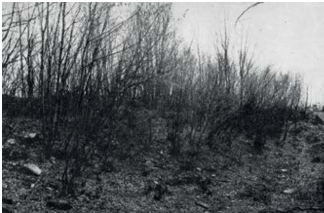
Figure 4. Medvedgrad castle before the conservation works in 1979
