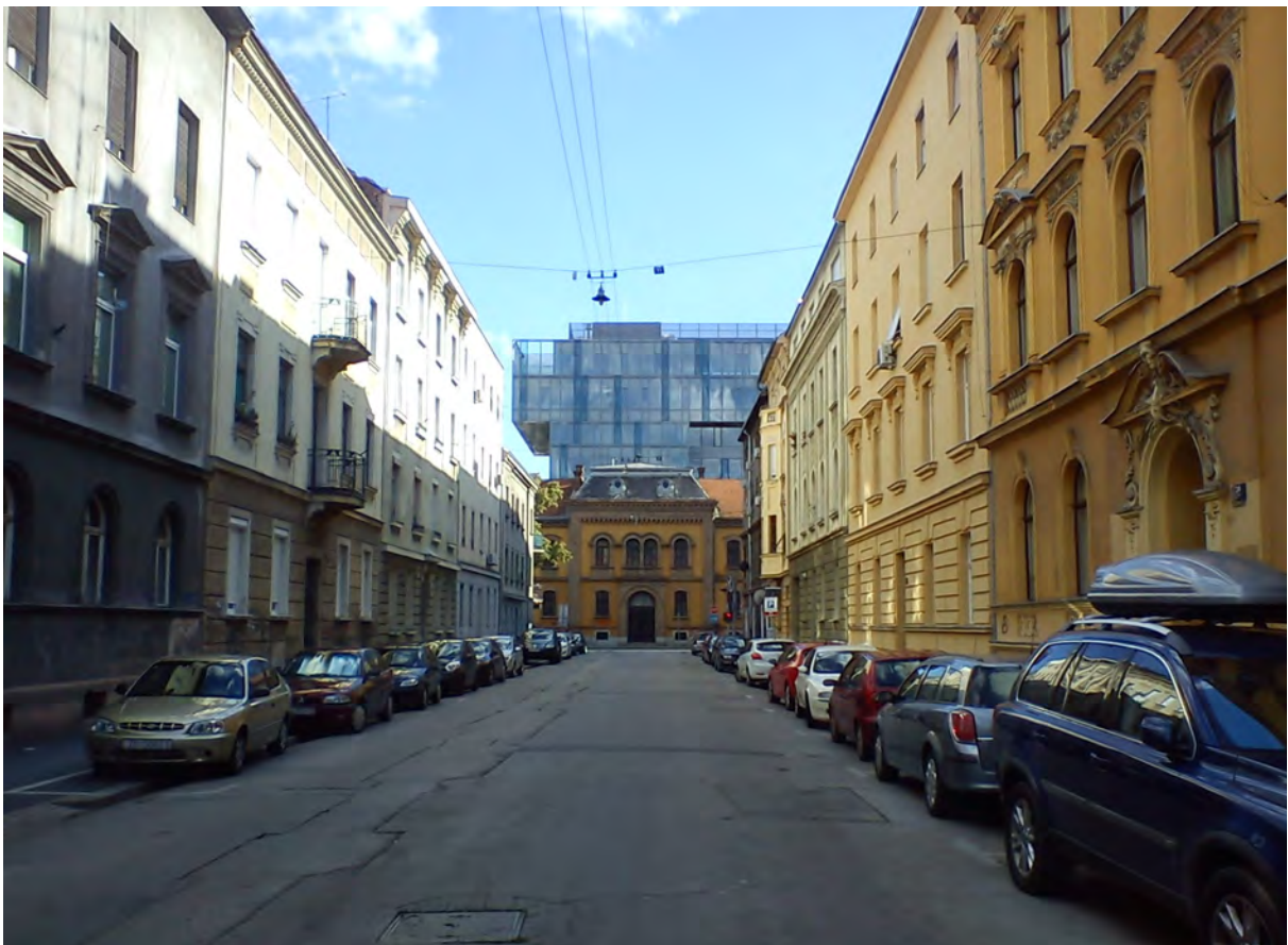
Fig. 1 What’s behind the corner?
