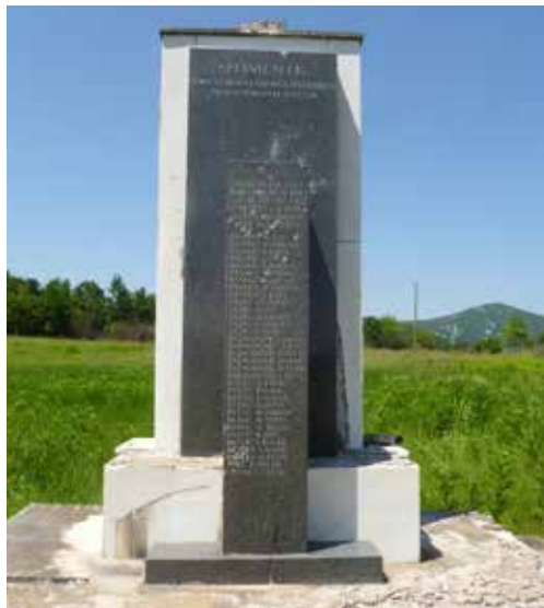
Figure 2. Damaged monument in Barlet, near Gospić
