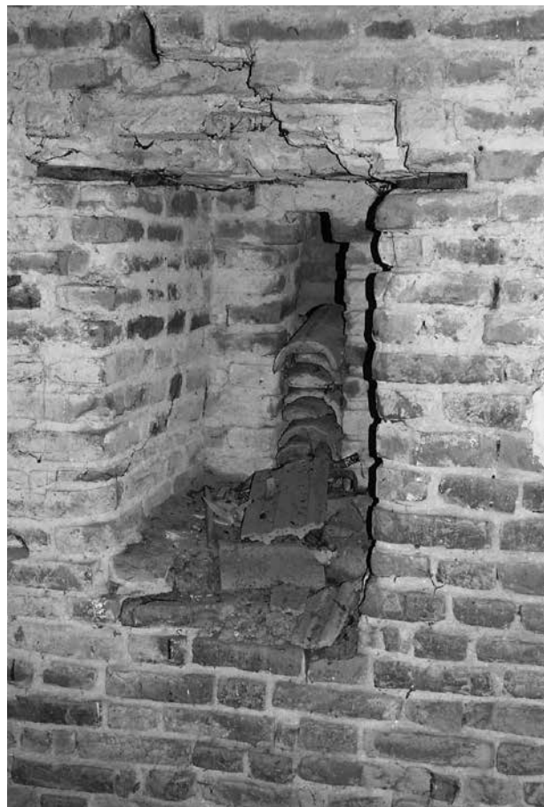
6. Kloštar Ivanić, crkva sv. Marije, zvonik, prvi kat, istočni zid, prozorski otvor (foto: M. Cepetić Rogić) / Kloštar Ivanić, church of St Mary, belfry, first floor, eastern wall, window opening (photo: M. Cepetić Rogić)
