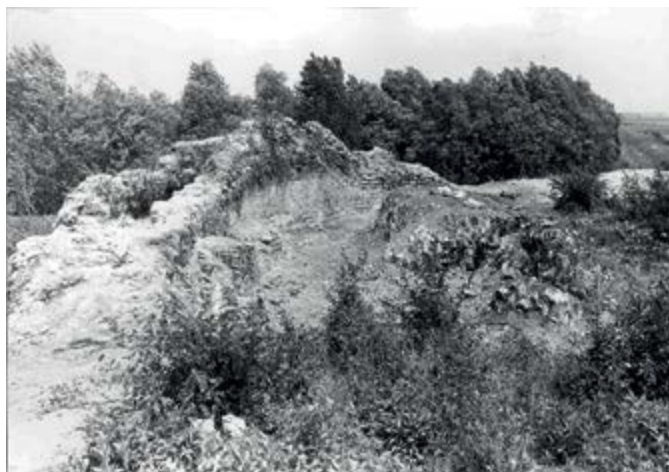
Figure 3. Clearance works at Kolodvar castle in 1967
