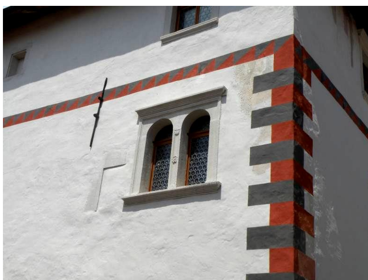
Fig. 9 Renaissance bifora on central pentagonal tower (photo: Tea Gudek Šnajdar).
