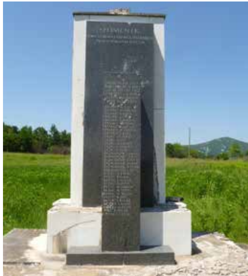
Figure 2. Damaged monument in Barlet, near Gospić
