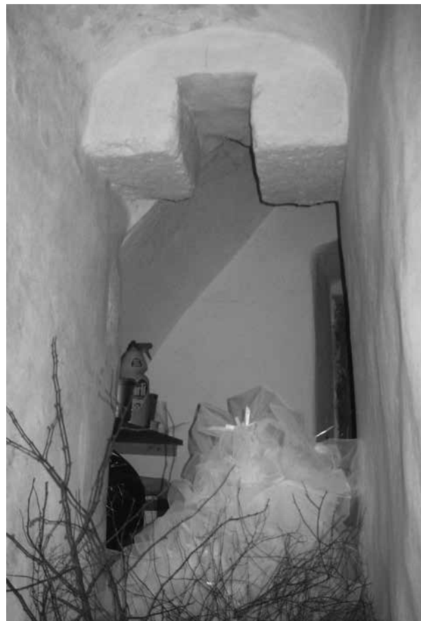
4. Kloštar Ivanić, crkva sv. Marije, zvonik, prizemlje, istočni zid, izvorni ulaz (foto: M. Cepetić Rogić) / Kloštar Ivanić, church of St Mary, belfry, ground floor, eastern wall, original entrance (photo: M. Cepetić Rogić)
