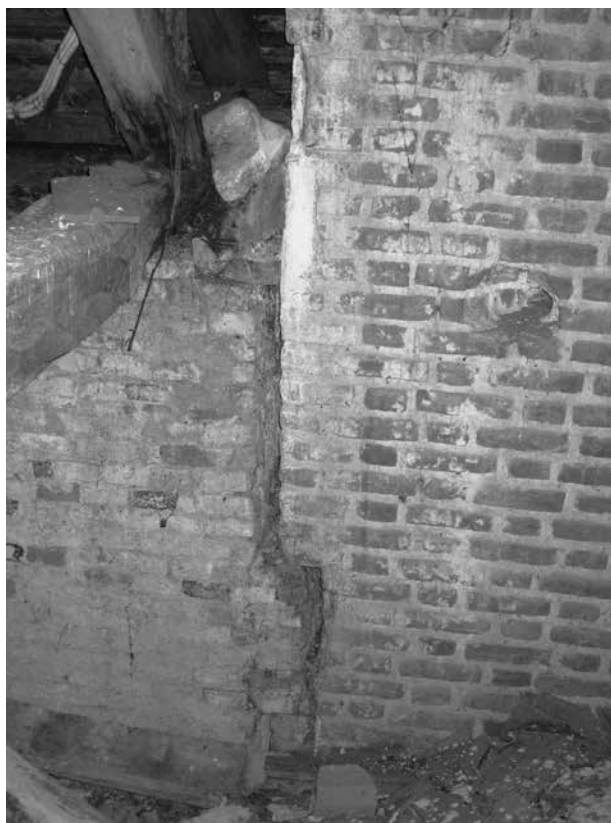
2. Kloštar Ivanić, crkva sv. Marije, tavan, pogled na zapadnu rešku između južnog zida zvonika i sjevernog zida broda (foto: M. Cepetić Rogić) / Kloštar Ivanić, church of St Mary, attic, view of the western seam between the southern belfry wall and the northern nave wall (photo: M. Cepetić Rogić)
