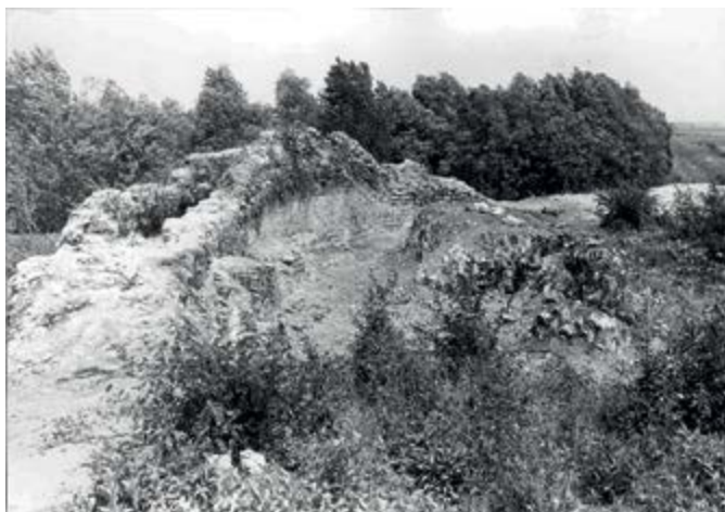
Figure 3. Clearance works at Kolodvar castle in 1967
