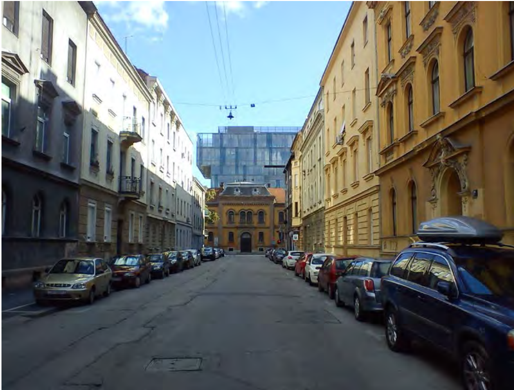
Figure 33. Zagreb, Primorska Street. What's around the corner?
