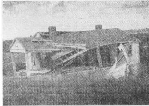
(2.) The wrecked, six-room, framed dwelling valued at around $5,000.00. Six sticks of dynamite did it. The house was blown to bits except for the foundation and the walls. KKK notes have threatened the Matthews, he house was built in a so-called "white only" community. However U. S. Judge Clarence Mullins on July 31 kicked that zoning law out. Police—city and county—say they can't find the dynamiters, as yet.
